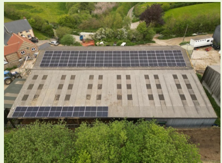
Solar Panels on a Farm Building Roof
