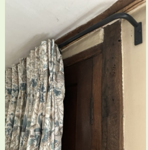
'French' curtain pole and thermal lined curtain
