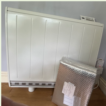
Quantum Heater and Reflective Heat panel (to be fitted)
